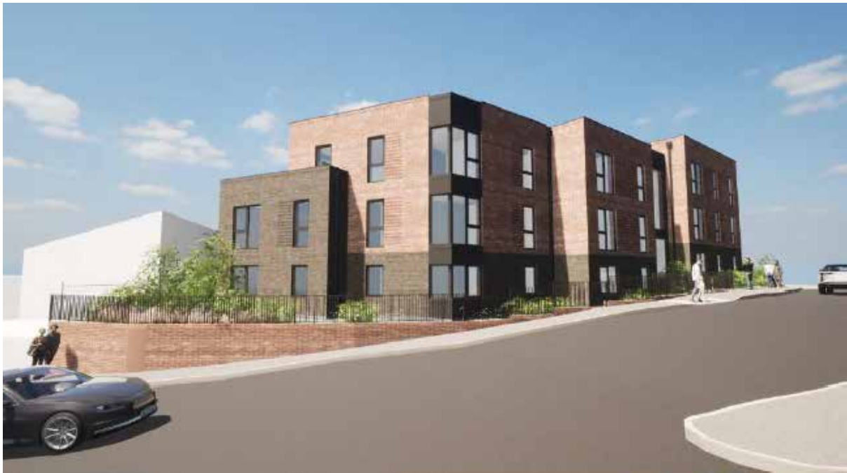
Corner elevation fronting Kelham Way junction
